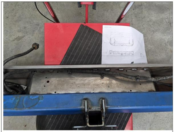
19. Fit the harness to the rear bar, routing the cables through the side arms so that the sensor wiring positions are in the correct locations.
